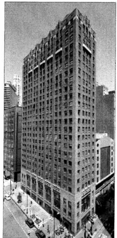
The Old Dearborn Bank Building in 2003.
